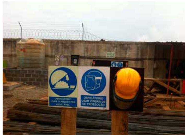
At the time of the HRIA in Angola (2011), 64 people were working on the Nestlé construction site.
