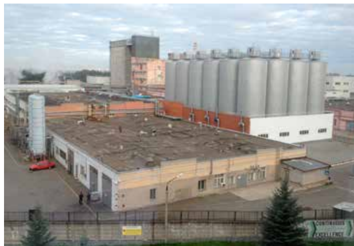
View over the industrial zone where the Nestlé Timashevsk factory is located, Russia
