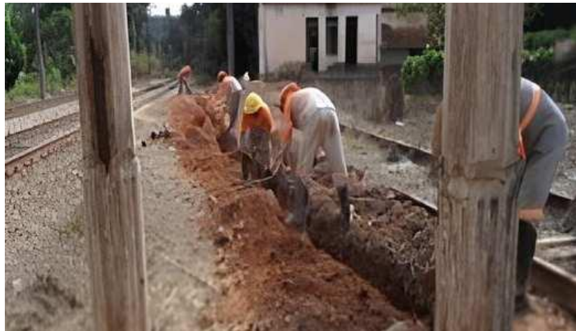
Figura 5 – Workers digging to repair railway signaling cables
