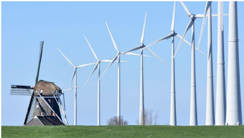
Figura 1 – Moinho e parque eólico. Retirada de https:// windcycle.energy/ windmill-vs-wind-turbine/ .
